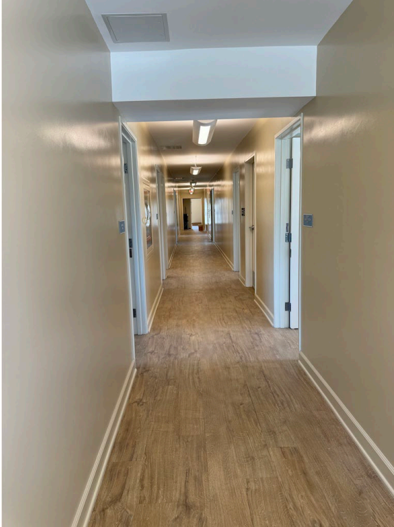
Photo 19 Main Building, second floor, corridor, view facing south
